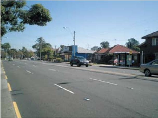
**FIGURE 3.3** SIGNIFICANT URBAN UNDIVIDED ARTERIAL ROAD (WITH DIRECT DRIVEWAY ACCESS)
