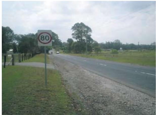
**FIGURE 3.7** UNDIVIDED RURAL ROAD WITH LESS THAN 5.6 METRES SEALED PAVEMENT
