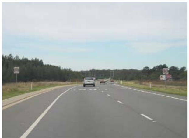
**FIGURE 3.10** RURAL UNDIVIDED ROAD WITH SEALED PAVEMENT GREATER THAN 5.6 METRES
